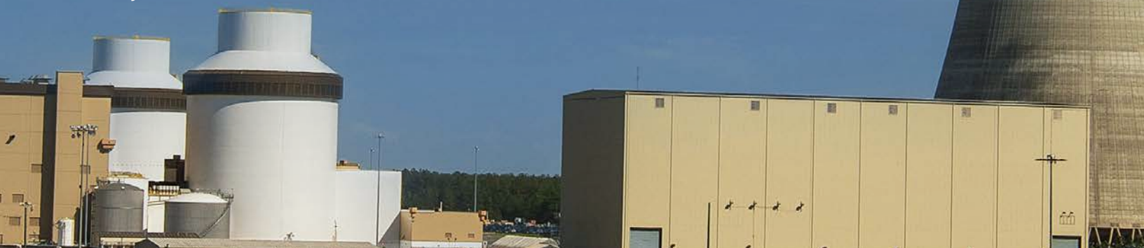
Plant Vogtle Units 3&4
