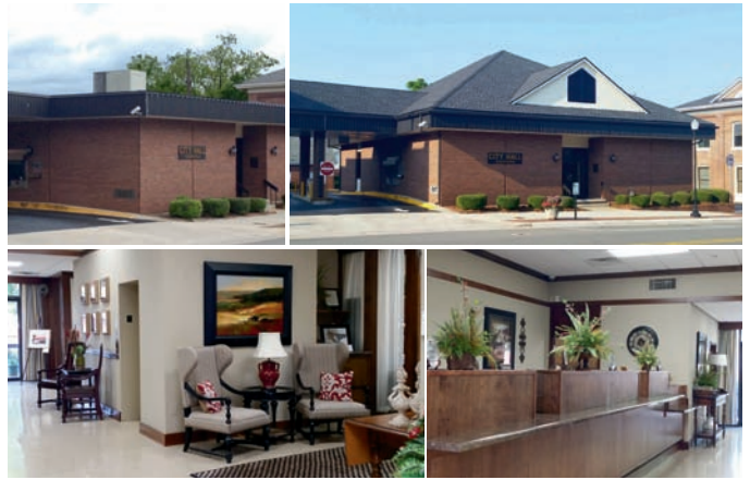
Top: Sandersville City Hall roof 'before' and 'after' Bottom: new lobby design and furnishings
